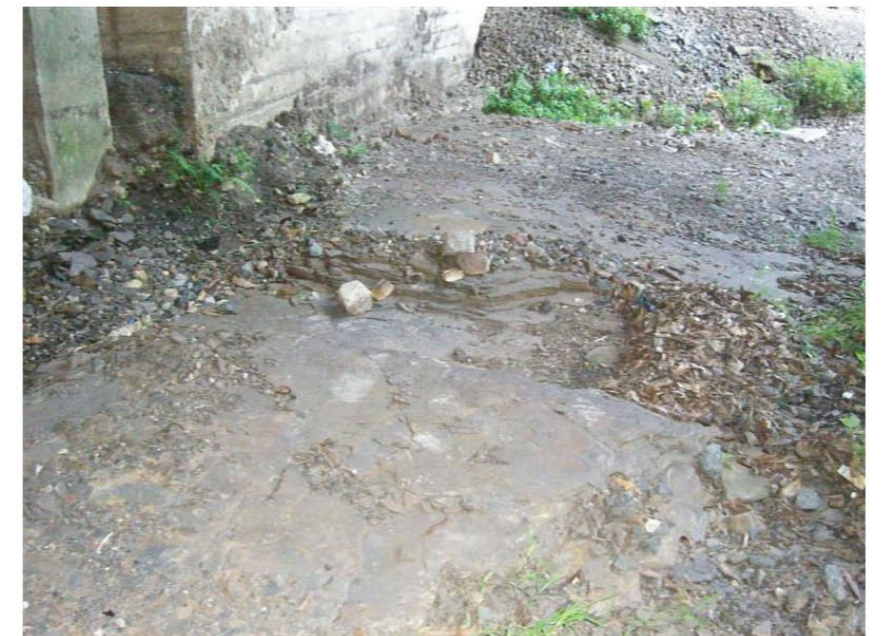
14. Exposed shale at base of excavation adjacent to Platform 11.
