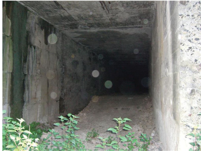
11. Up Southern Suburbs "tunnel" looking from the void away from Sydney. Note that a considerable quantity of spoil from track reconditioning has been placed in the tunnel.
