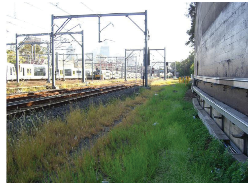
2. Down side of rail corridor looking towards Central from the Sydney side of Lawson St Overline bridge
