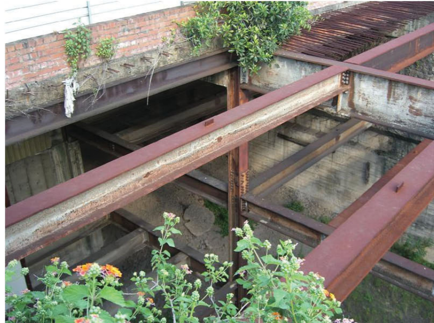
23. From the car park looking towards the start of the Up Southern Suburbs tunnel.
