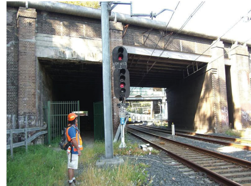
1. Lawson St Overbridge - Sydney Face showing portal of Down Southern Suburbs Railway dive adjacent to the Down Illawarra Line. Note that the cable troughs on the wall are marked High Voltage and probably contain RailCorp 11kV feeders 539 and 620/2
