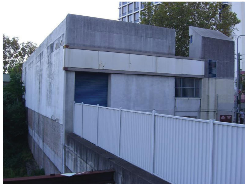
20. From the car park looking towards Sydney at the entrance building for platforms 11&12.
