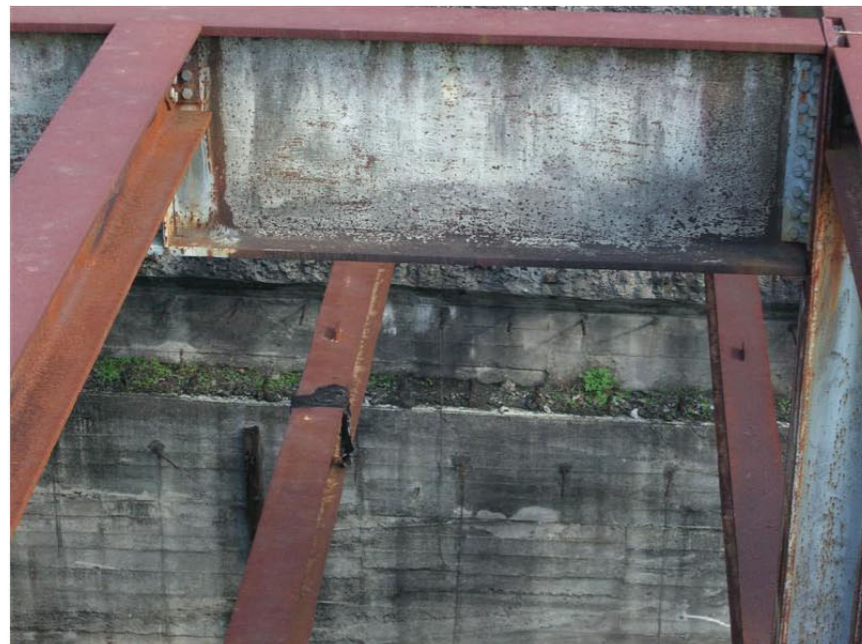
24. From the car park looking across to void towards platform 10.
