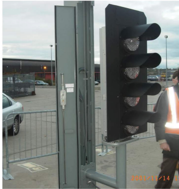
Figure 20 - Close up of Gatsometer BV height adjustment system
