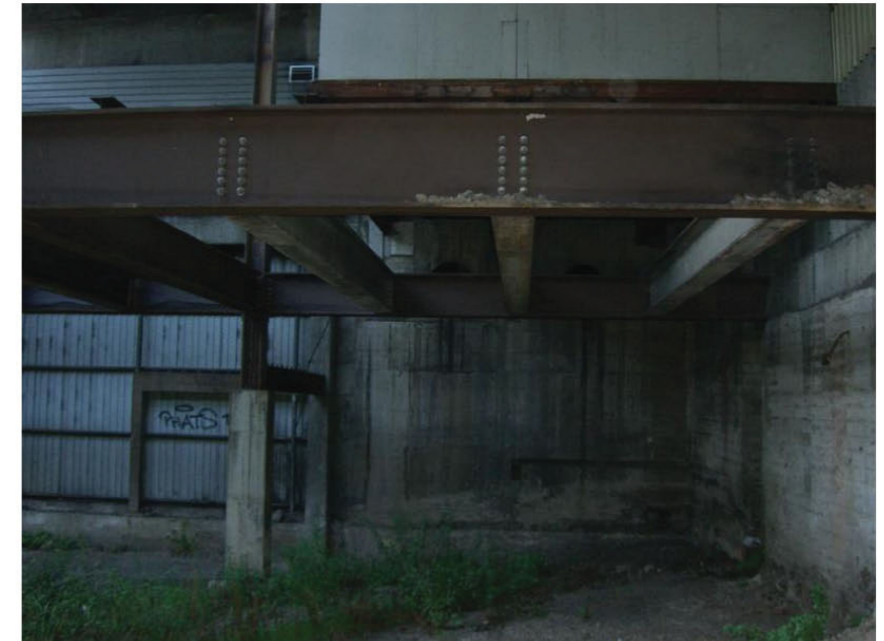
13. Steel beams within the void.
