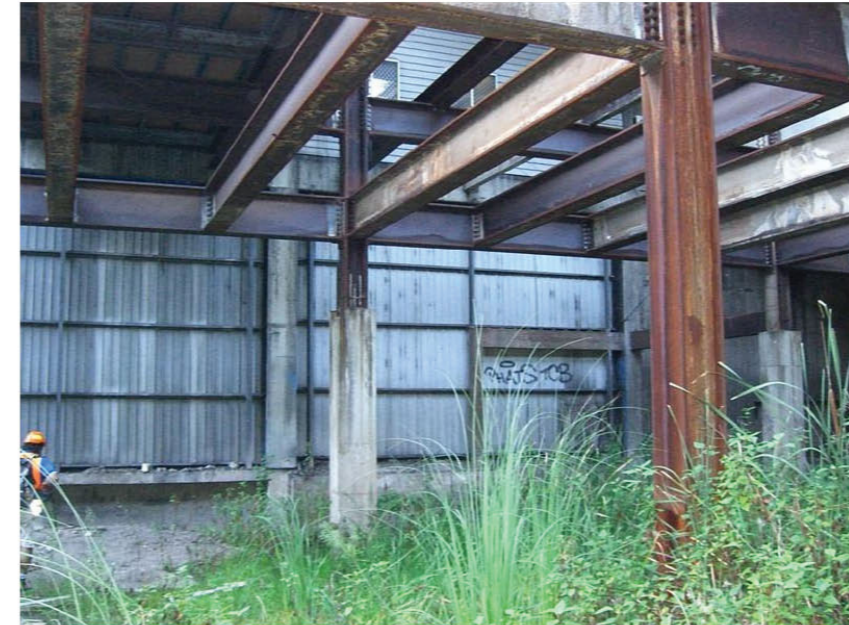
9. Sheet steel wall between void and platform 11
